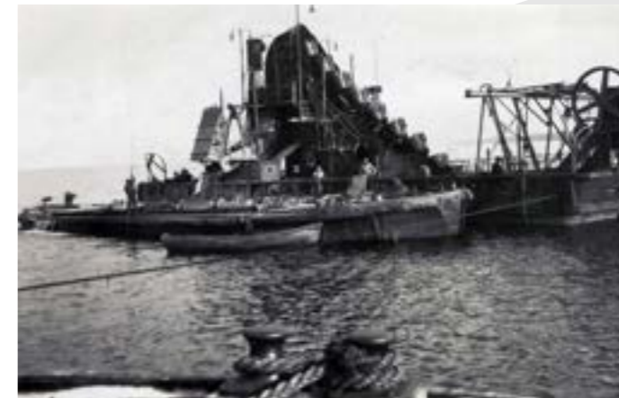
Special machinery equipped with buckets was used in digging the Karosta Canal.
